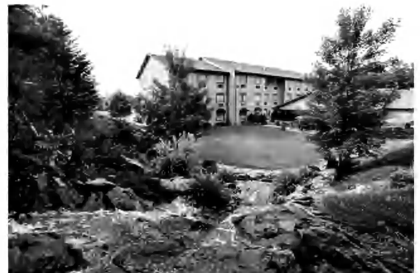
Mountain Lodge and Conference Center
